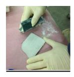
Sand any bonding surfaces where the endcap is to be installed (including on the gutter).
