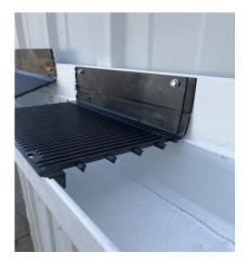
To apply leaf guard to G-90 (4x6) if there is enough facia above the gutter exposed you can apply the leaf guard and screw through the leaf guard flange into the facia board. If you do not have the facia height or the drip edge is in your way you can rip the leaf guard using a saw. And angle screws at back of gutter into facia
